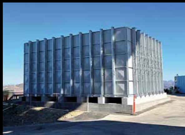
OUTDOOR TANK WITH STEEL SKID FOOTING
